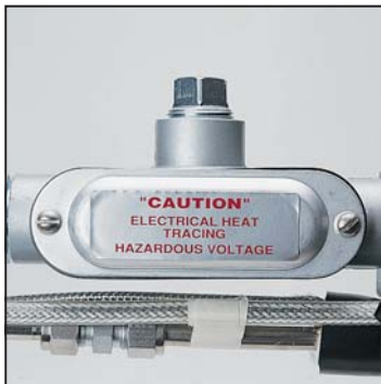
Assembled Input Power and Splice Connection Kit
